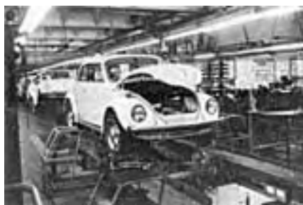
The final assembly line. These U.S. Spec. models have different headlamps, bumpers, front flashers and a slotted apron for air conditioning.
