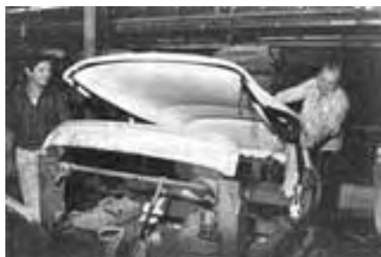
In a workshop a few hundred yards away, skilled craftsmen are constructing the folding roof on a jig.
